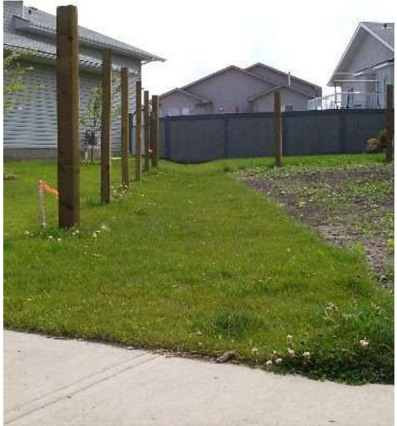
The result of a well-planned and properly executed grading and surface drainage system is a lot free of ponding, with no adverse effects to adjacent properties.
